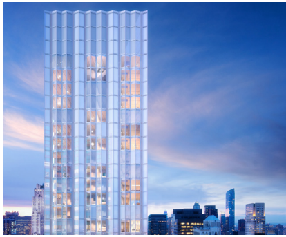
100 East 53rd Street
